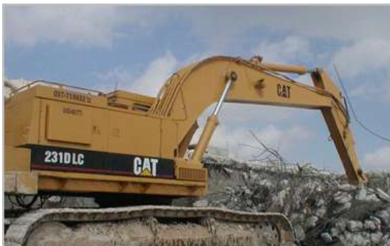
Image 20 Bulldozing a house
