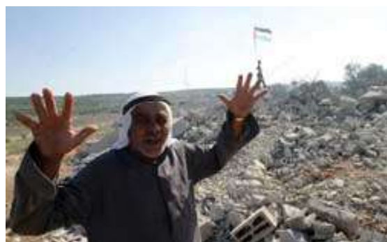
Image 21 House demolition in Abu Tur
