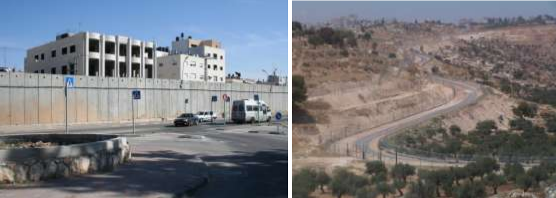
Images 9 - 10: Components of the Segregation Wall: Concrete Panels, Barbed Wires,
