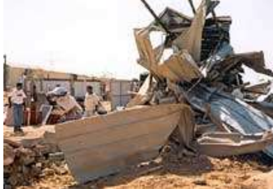
Image 2 Demolished House near Beer Sheva
