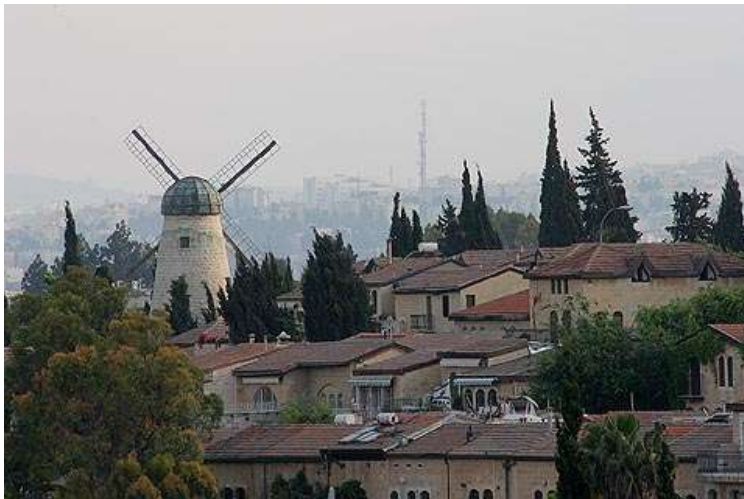
Image 12 Windmill Quarter today, renovated, - view to the western new city
